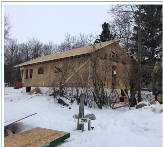
More new home construction underway, 2021
